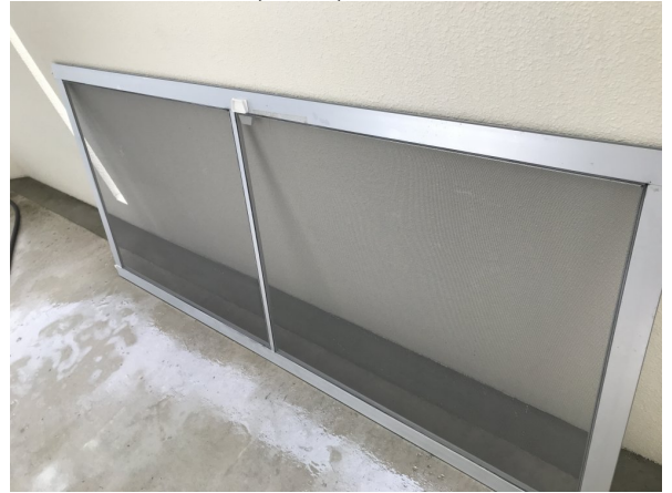
14.網戸張り替え (after)
