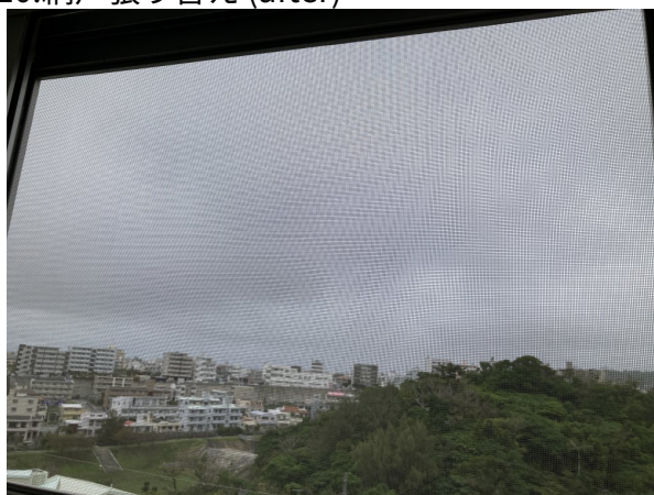
10.網戸張り替え (after)
