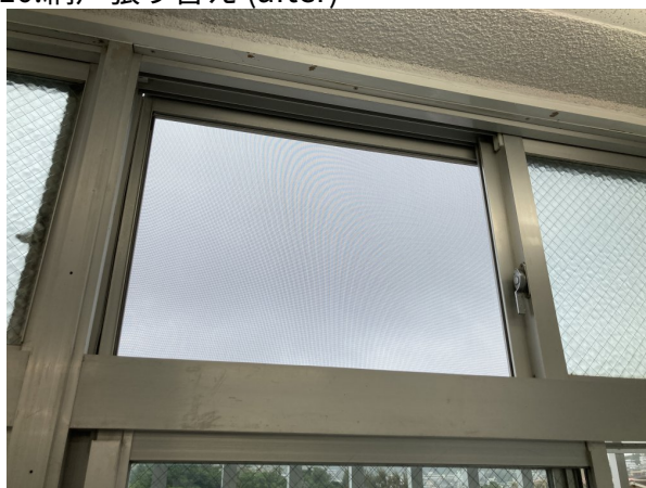
10.網戸張り替え (after)
