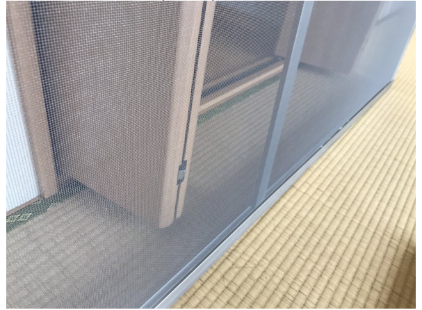
16.網戸張り替え (after)
