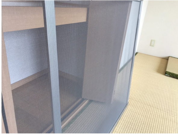
16.網戸張り替え (after)
