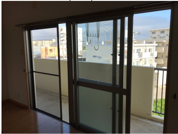
16.網戸張り替え (after)
