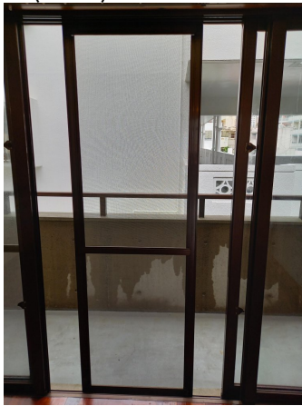
16.網戸張替 (after)
