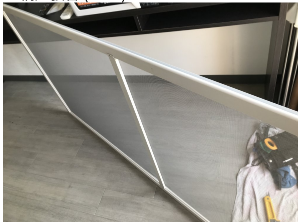
11.網戸張替 (after)
