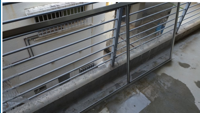
17.網戸張替 (after)
