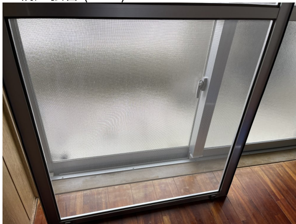
13.網戸張替 (after)
