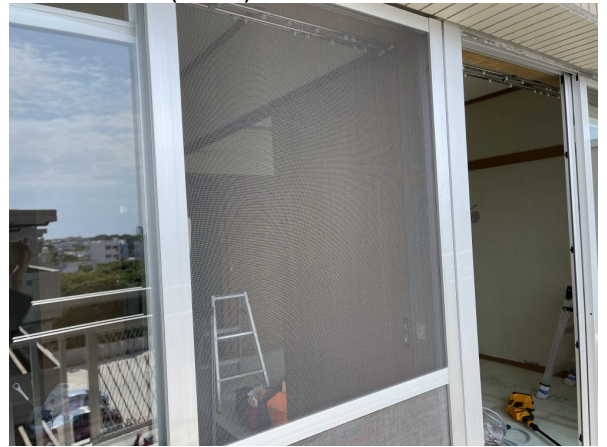
13.網戸張替 (after)
