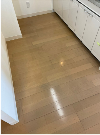
23.床剥離洗浄before
