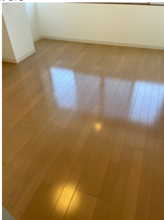
23.床剥離洗浄before
