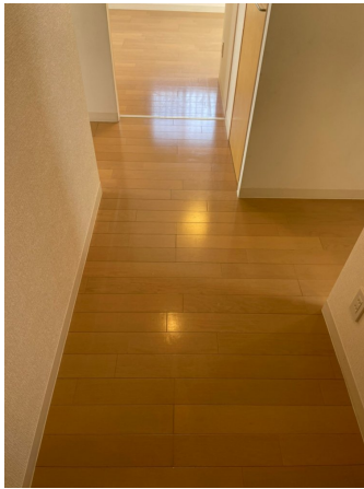
23.床剥離洗浄before
