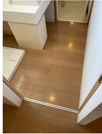
23.床剥離洗浄before
