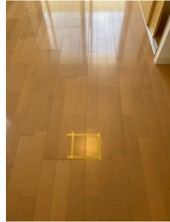
23.床剥離洗浄before
