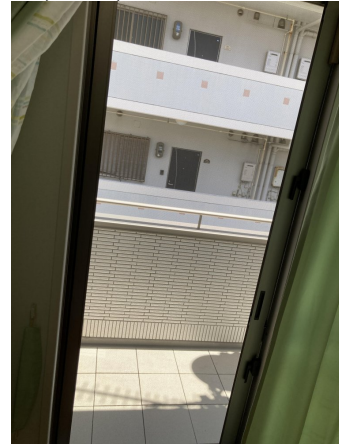
20.網戸張替 (after)
