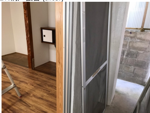
17.網戸張替 (after)
