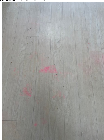
21.床剥離洗浄before
