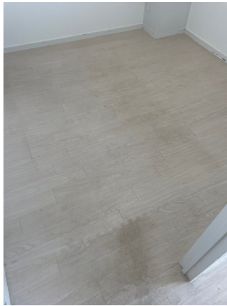
21.床剥離洗浄before
