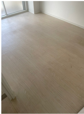
21.床剥離洗浄before
