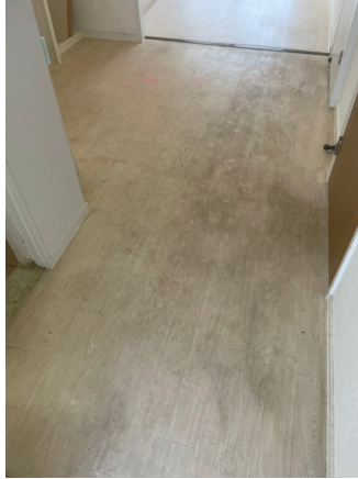
21.床剥離洗浄before
