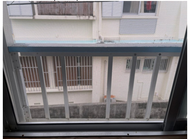
14.網戸張替 (after)
