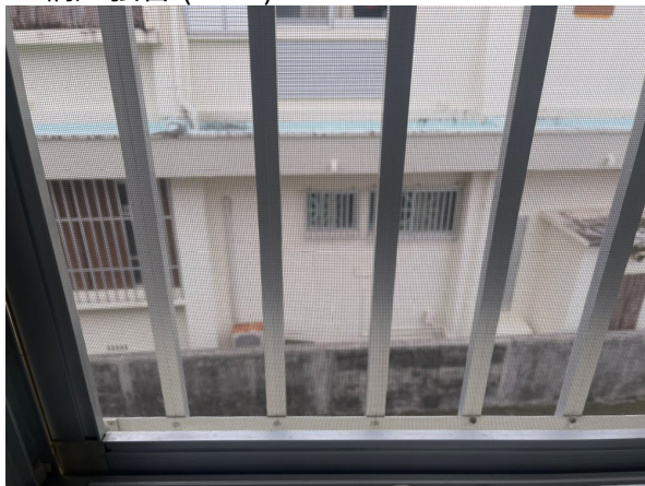
14.網戸張替 (after)
