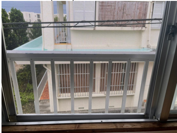
14.網戸張替 (after)
