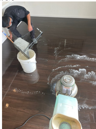
16.床剥離洗浄before
