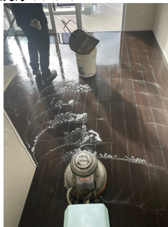
16.床剥離洗浄before
