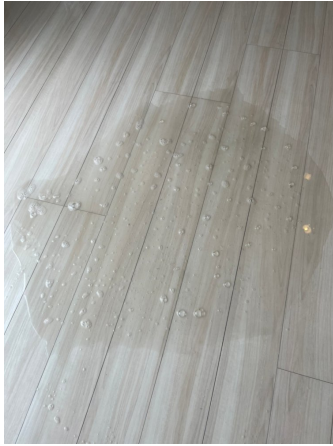
19.床剥離洗浄before
