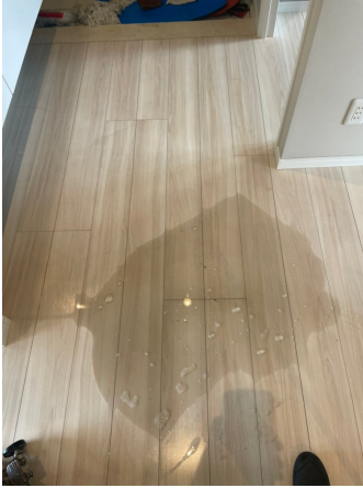
19.床剥離洗浄before
