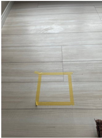
19.床剥離洗浄before
