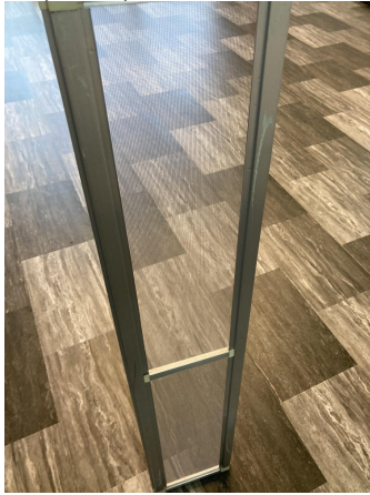
14.網戸張替 (after)
