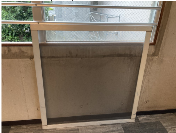
14.網戸張替 (after)
