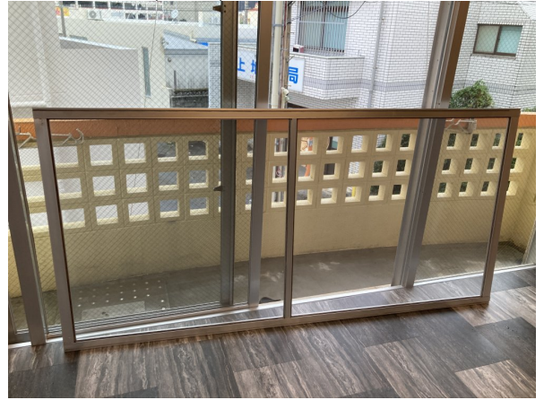
14.網戸張替 (after)
