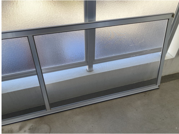
16.網戸張替 (after)
