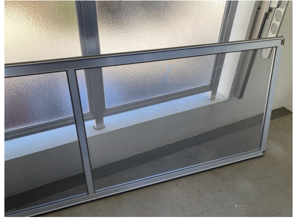
16.網戸張替 (after)
