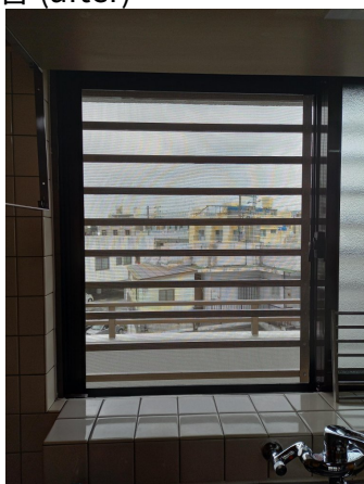
18.網戸張替 (after)
