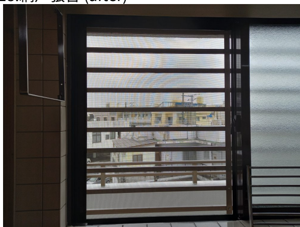
18.網戸張替 (after)
