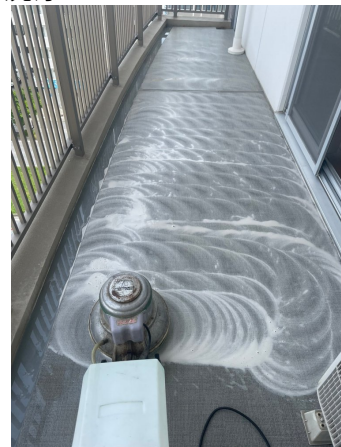
33.床剥離洗浄before
