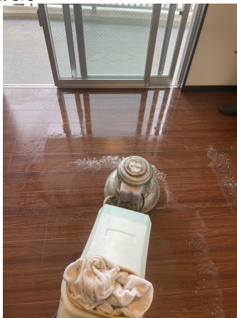
33.床剥離洗浄before
