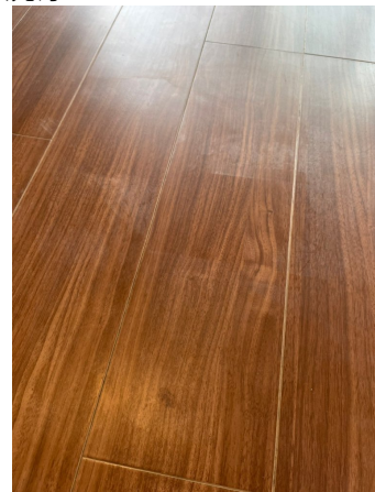
33.床剥離洗浄before
