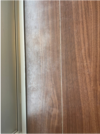
33.床剥離洗浄before
