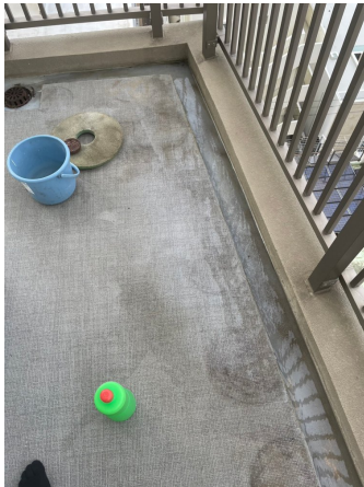
33.床剥離洗浄before
