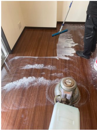
33.床剥離洗浄before
