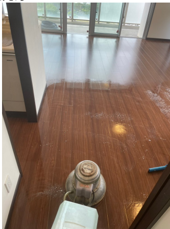
33.床剥離洗浄before
