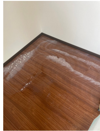
33.床剥離洗浄before
