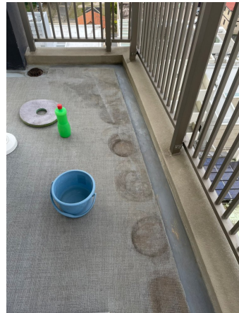
33.床剥離洗浄before
