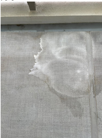
33.床剥離洗浄before
