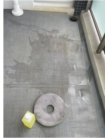
33.床剥離洗浄before
