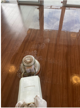
33.床剥離洗浄before
