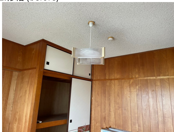
照明取替before
