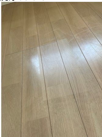
22.床剥離洗浄before
