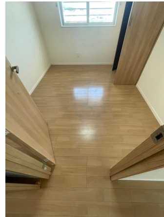
22.床剥離洗浄before
