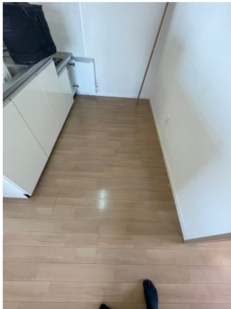
22.床剥離洗浄before
