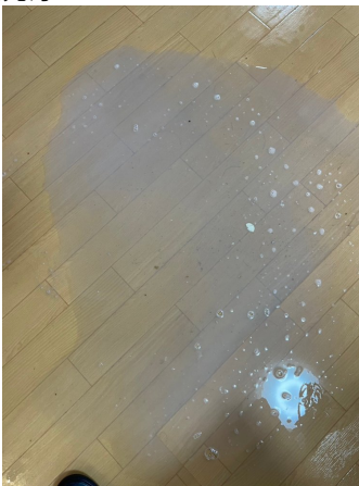
15.床剥離洗浄before
