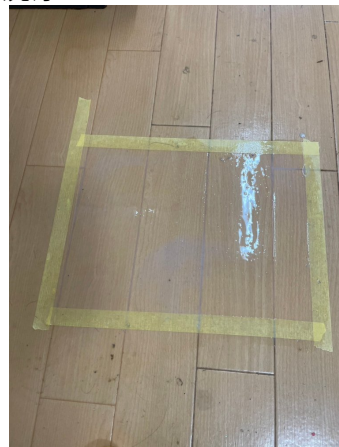
15.床剥離洗浄before
