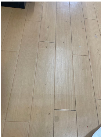
15.床剥離洗浄before
