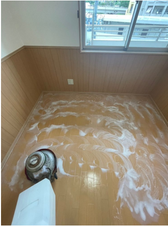
15.床剥離洗浄before
