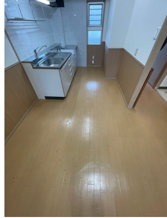
15.床剥離洗浄before
