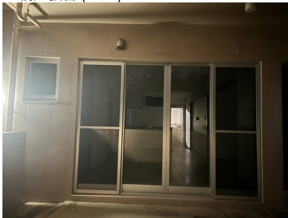
18.網戸張替 (after)
