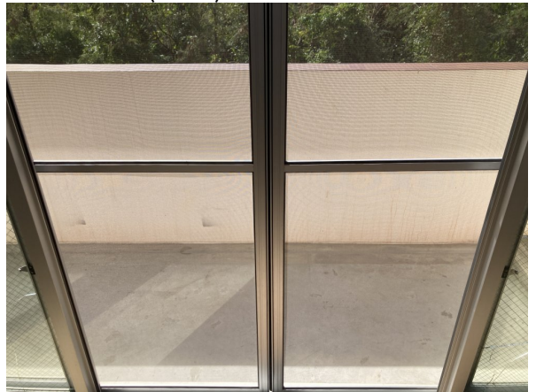
17.網戸張替 (after)
