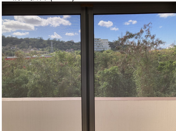
17.網戸張替 (after)
