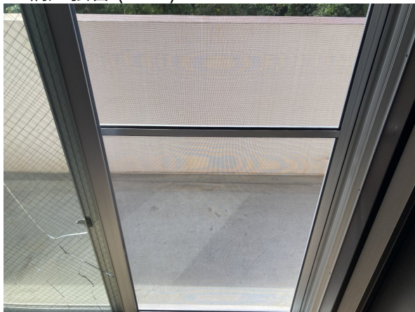
17.網戸張替 (after)
