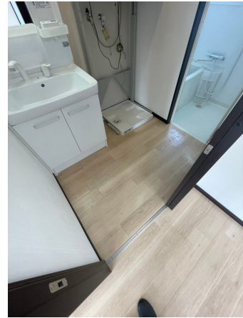
18.床剥離洗浄before
