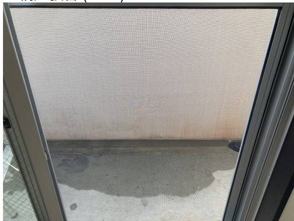
17.網戸張替 (after)
