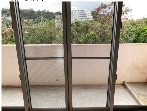
17.網戸張替 (after)
