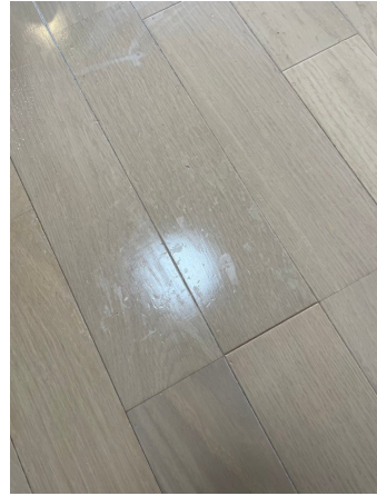
23.床剥離洗浄before
