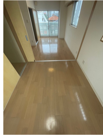
23.床剥離洗浄before
