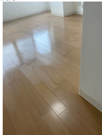
23.床剥離洗浄before
