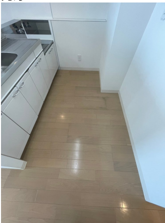
23.床剥離洗浄before
