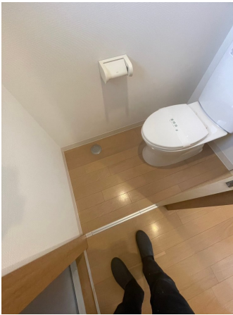
23.床剥離洗浄before
