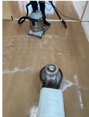
23.床剥離洗浄before
