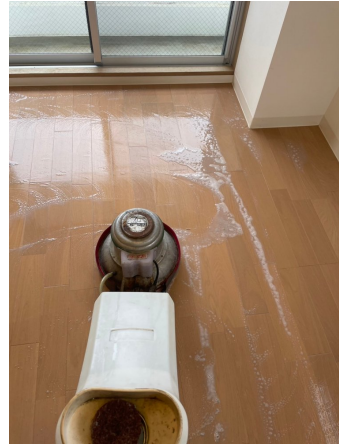
23.床剥離洗浄before
