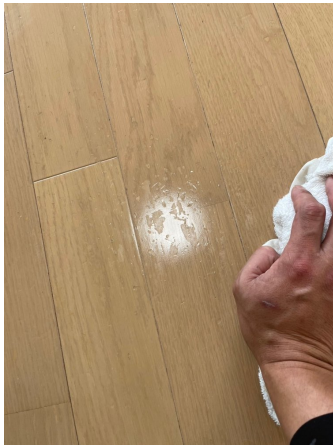
23.床剥離洗浄before
