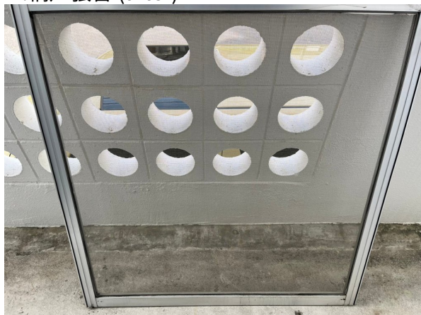
17.網戸張替 (after)
