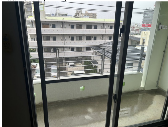
2.網戸張替 (after)
