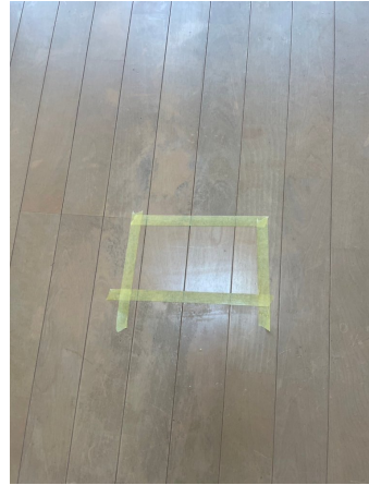
16.床剥離洗浄before
