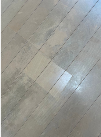
16.床剥離洗浄before
