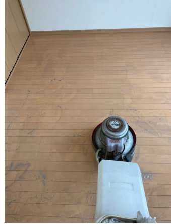
16.床剥離洗浄before
