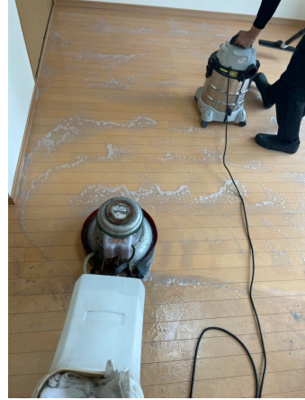
16.床剥離洗浄before
